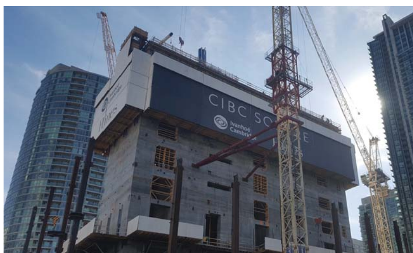
Figure 2: Three Luffing Cranes in the Foreground and Background at CIBC Square [8]
